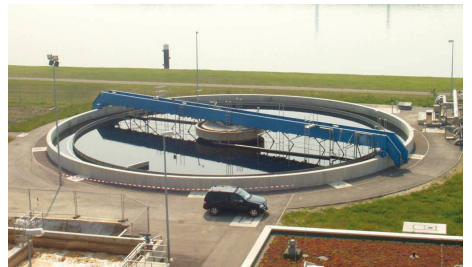
▪ HIK Doppel-Rundschildräumer / HIK double circular-tank shield scraper
