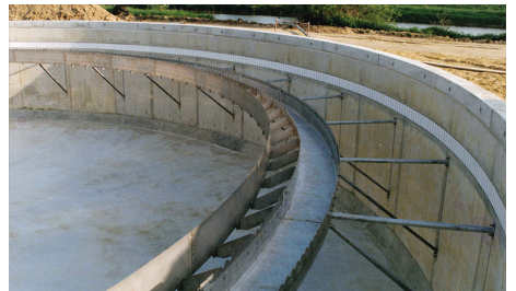
▪ HIK Klarwasser-Ablaufrinne / HIK double-sided clear water channel
